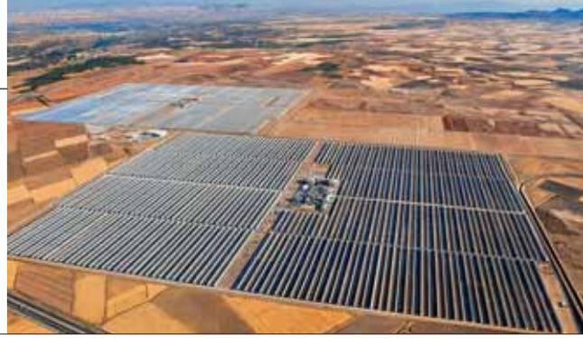
**Andasol 1 + Andasol 2 – Two 50 MW Parabolic Trough Power Plants with Storage, Spain**
