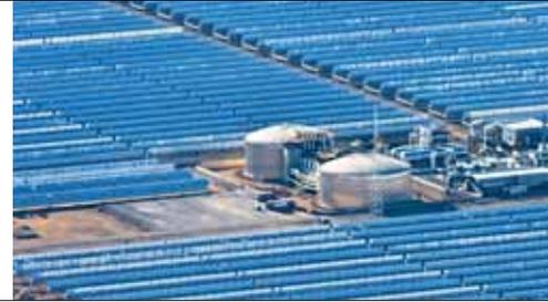
Parabolic Trough Power Plant with Thermal Storage
